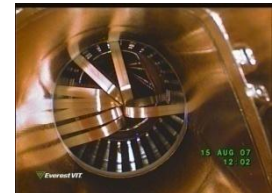
A plug-in module (right) damaged during a cool-down/warm-up thermal cycle of the magnets
